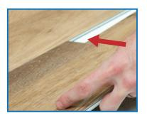
Slide the plank along the short side until it reaches the long side of the previous row of planks.
