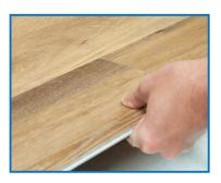
Drop gently. During the fold down, make sure the planks are tight against each other. Press with your palm on both ends of the plank. Planks are now fully locked.
