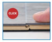
Press with your thumb on both ends of the short side. Continue pressing until you hear the "click" sound of the lock system.
