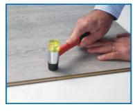
Hit gently with a soft-face mallet on both sides of the short end. Planks are now fully locked.
