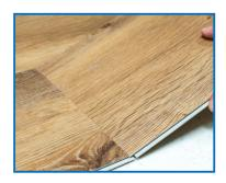
Start by engaging the plank on the short side with the installed plank.
